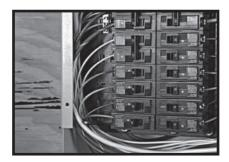
Each wire in the pre-wired transfer switch is color-coded so you can easily match circuits in the main panel to their new breakers in the transfer switch.
